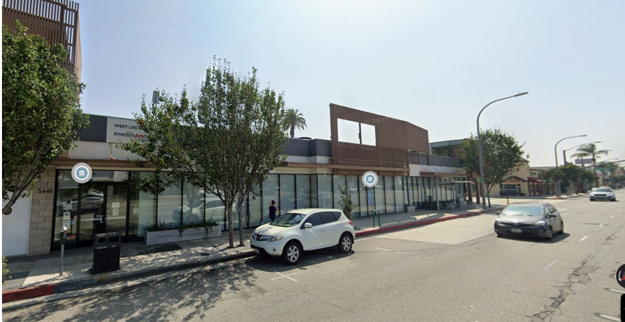
5446 Sepulveda Blvd. building entrance on Sepulveda
